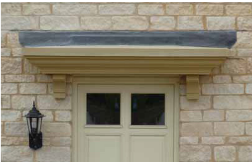
Figure 1: GRC door canopy used with Cotswold stone.
